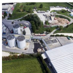
Anaerobic Digestion plant in Bassano del Grappa (approx. 1h 30 mins from Venice)
