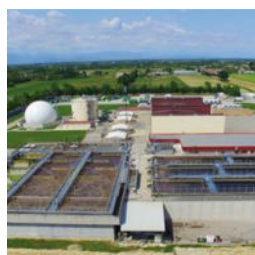
Bio Treatment plant in Camposampiero (approx. 1hr from Venice)
